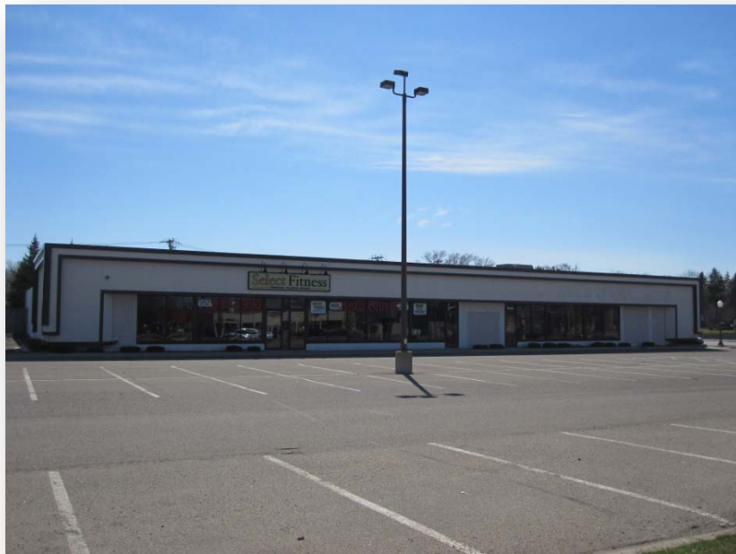
Vacant strip mall located at the southeast corner of Shady Oak Road and Excelsior Boulevard.
