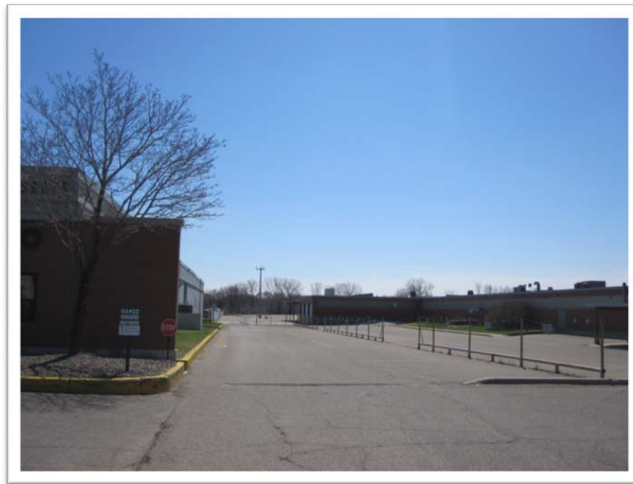
Surface parking between NAPCO (left) and the Hopkins Tech Center (right). Station platform will be located directly behind the Hopkins Tech Center.
